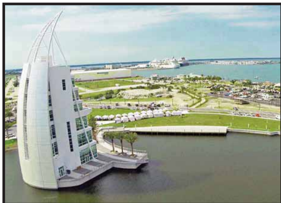
Vista de Exploration Tower .
